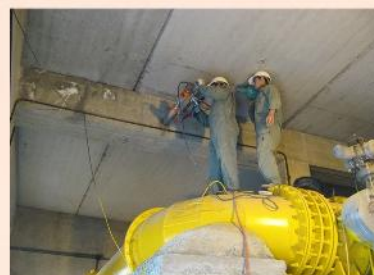
▲ Z.J Engineering technician using coring machine
