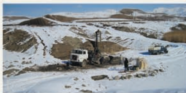
▲ Exploration drilling, Spiran bridge site
