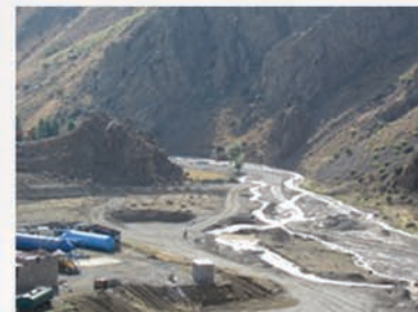
▲ Quality control of Earthwork operations
