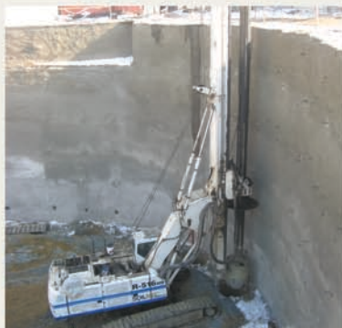
▲ Pile Installation, Tavrij Residential Tower
